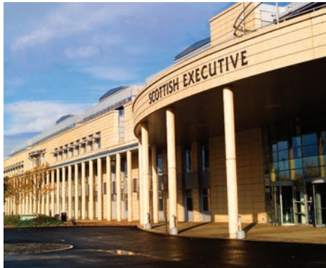
The Victoria Quay building became part of the Scottish Executive following devolution to the Scottish Parliament in 1999. It is the largest single office of the Scottish Government and contains Development and Education Departments.
